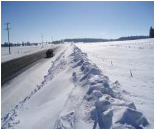
Snow removed from WA HWY 129 January 25, 2008. Snow bank > 10’ height. Tops of planted trees on right side of picture buried by drifting snow. Soon they will capture more snow and decrease drifting onto the highway.
